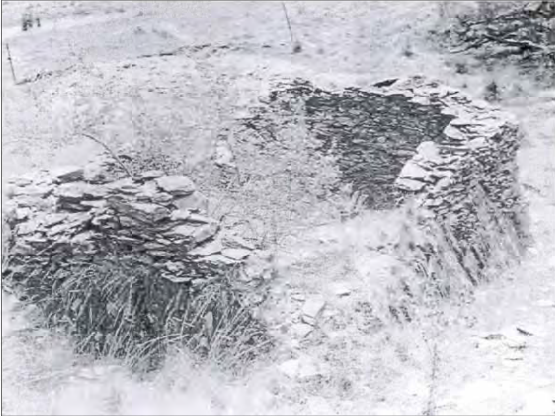
PLATE 3.8 1993 photograph of main stone structure, view to northeast
